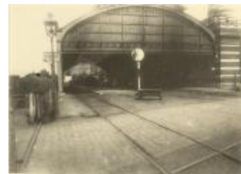
Station : overdekte spoorhal (Foto 04588_01 tem 04)
