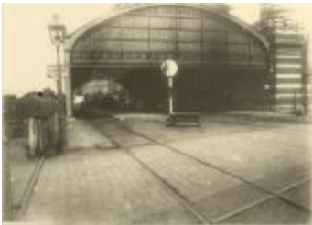
Station : overdekte spoorhal (Foto 04588_01 tem 04)
