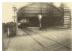
Station : overdekte spoorhal (Foto 04588_01 tem 04)
