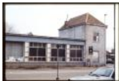
Covee (Dia container 21__52)
