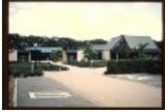
Crematorium (Dia's container 41_3622 + 26)
